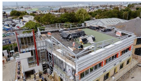
Figure 13: Installation of the Biosolar roof at East Kent College
